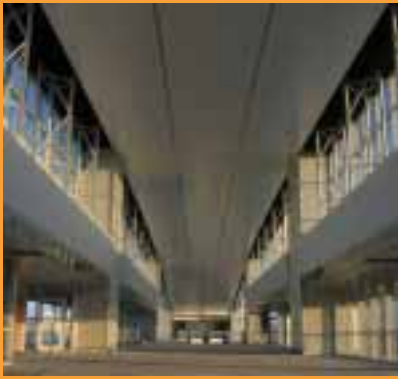
SkyLink Station - Platform level interior
