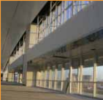
SkyLink Station - Platform level
